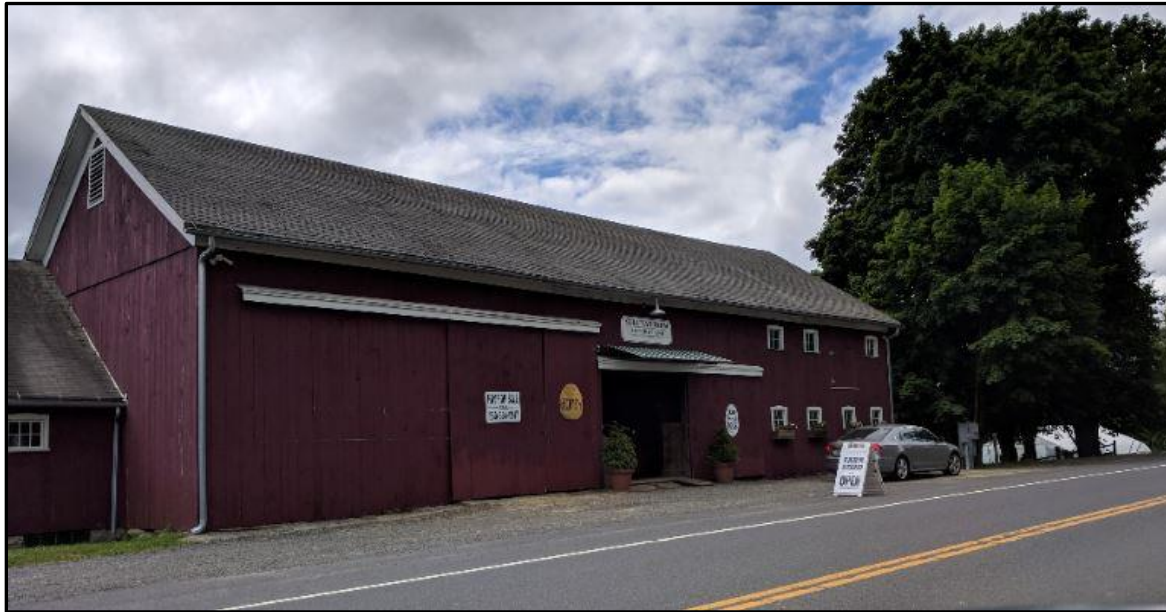
Photo 1 – view towards the south property line
