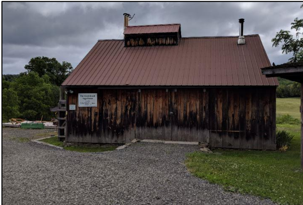
Photo #5: Access driveway, with sugar-house in background
